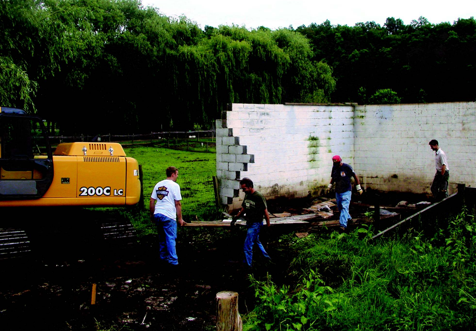
L-R: Frank Tiano, Jr., Cliff Cobrin, Frank Tiano, Sr. and Troy Gangle demolish the last original run-in shed on the property. The concrete block will be crushed and used as a base for our new pig barn.
