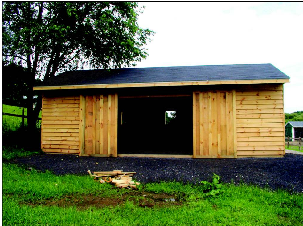
The new sheep barn -- almost finished in this photo!
